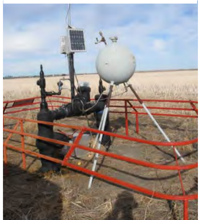
Figure 5: Methanol sphere installation
